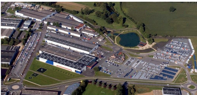
Gruau Group Headquarters
